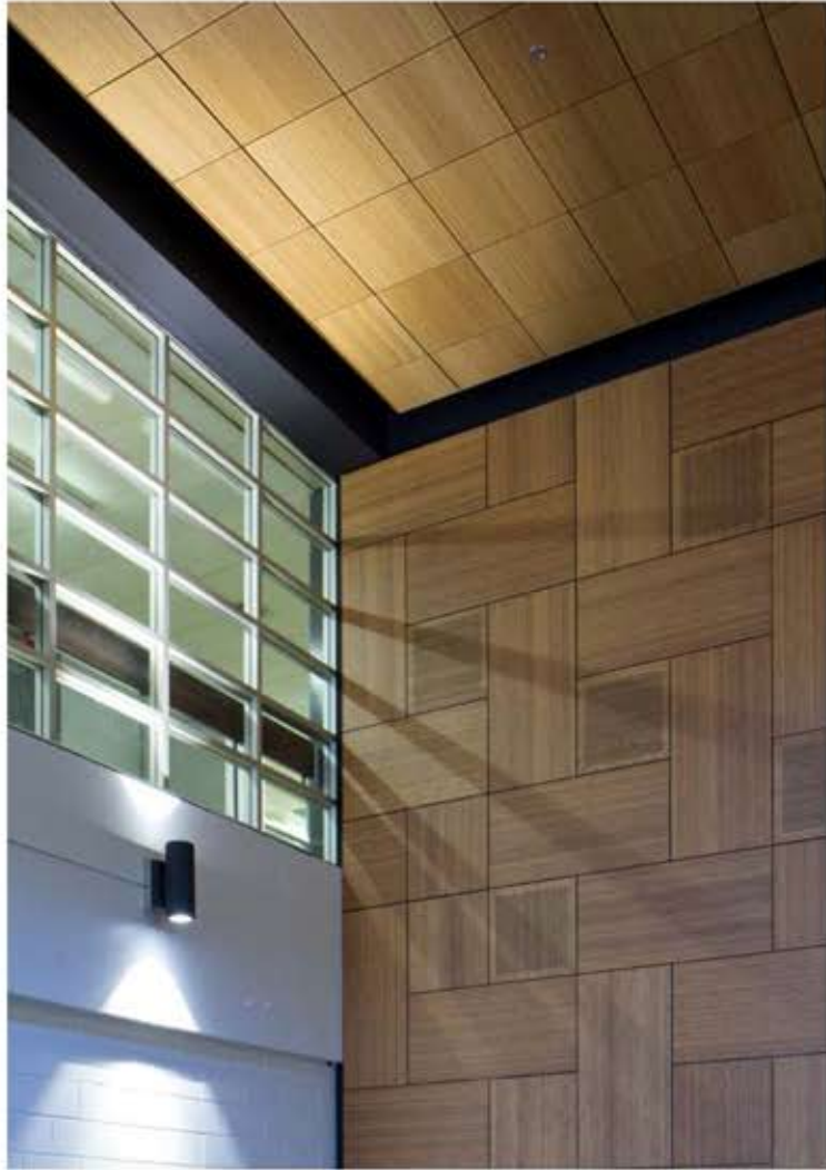
Products: Dry Internal F, Acoustic / Wood: Caramel Bamboo Ecole secondaire d'Anjou (Montréal, QC, Canada)
